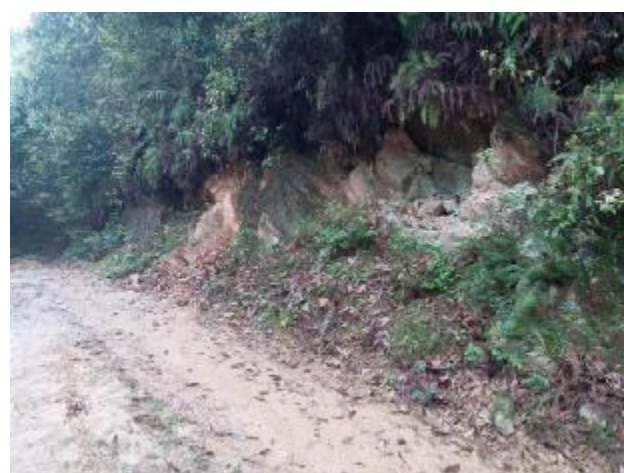
图2-5 土石路边坡板岩板理面较陡倾角45° (北部D7_N29° 19' 39.42" -E113° 16' 43.40")
