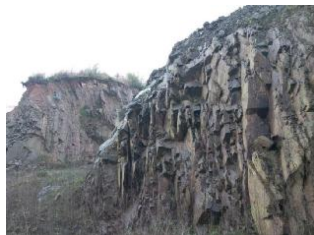
图2-4 挖方边坡板岩板理面产状10°∠80° (北部D5_N29° 19' 31.67" -E113° 16' 42.43")
